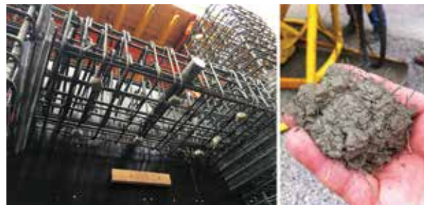
Figure 7. Kiara SFRC coupling beam.
