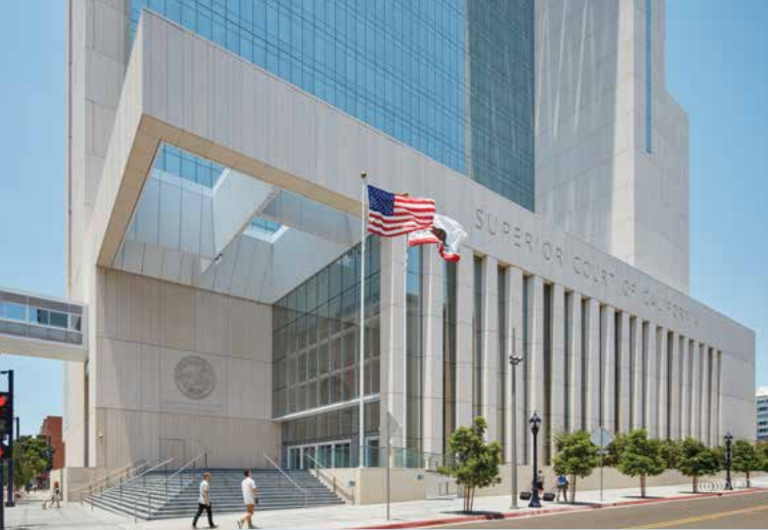
Figure 1. View of new San Diego Central Courthouse at the main entrance. Courtesy of Bruce Damonte.
