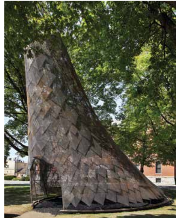
Pierce Engineers, Inc., was an Award Winner for its Wiikiaami project in the 2018 Annual Excellence in Structural Engineering Awards Program in the Category – Other Structures. Courtesy of Hadley Fruits.
