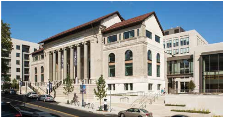
Silman was an Outstanding Award Winner for its University of Connecticut Downtown Hartford Campus project in the 2018 Annual Excellence in Structural Engineering Awards Program in the Category – Forensic/ Renovation/Retrofit/Rehabilitation Structures over $20M.
