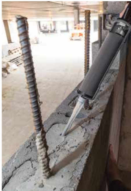
Bonding rebar into grouted concrete masonry walls.
