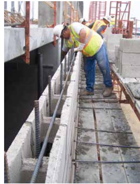
Figure 1. Reinforced concrete masonry construction.
