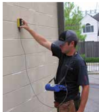
Figure 5. Locating vertical and horizontal masonry reinforcement with a pachometer.
