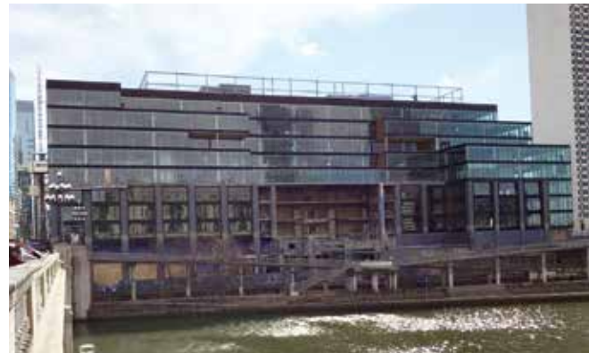
The Harman Group was an Award Winner for its Aramark Headquarters project in the 2018 Annual Excellence in Structural Engineering Awards Program in the Category – Forensic/Renovation/Retrofit/Rehabilitation Structures over $20M.
