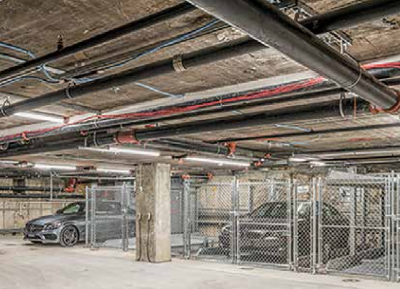
Beacon Street garage interior showing one of two interior columns.
