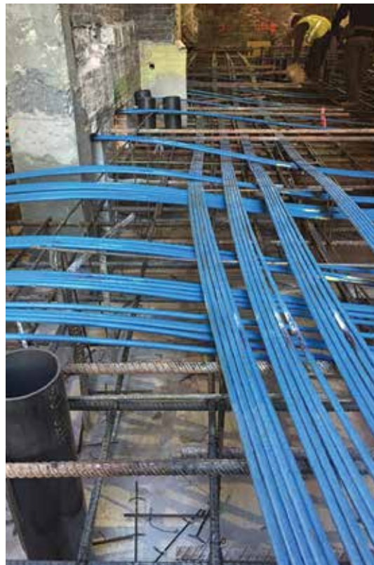
Interwoven post-tensioning tendons.
