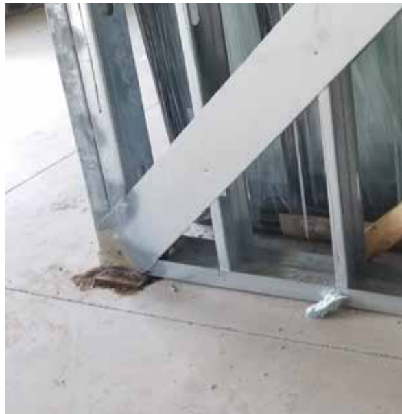
Figure 6. Steel embed in concrete at podium to CFS wall above.
