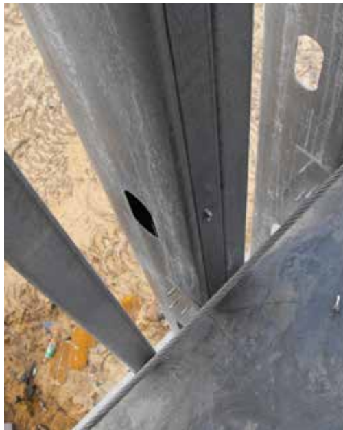
Figure 3. Nested jamb with studs and track.
