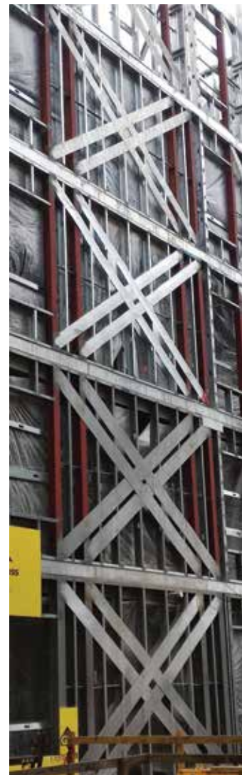
Figure 5. Overlapping shear straps for lateral resistance.
