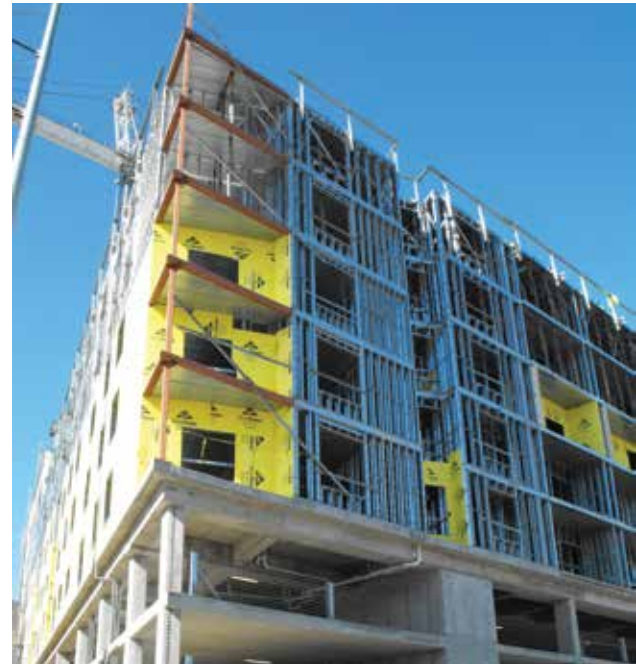
Figure 1. Concrete podium with CFS above.
