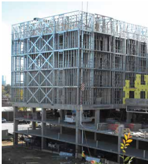
Figure 2. CFS over parking structure podium.
