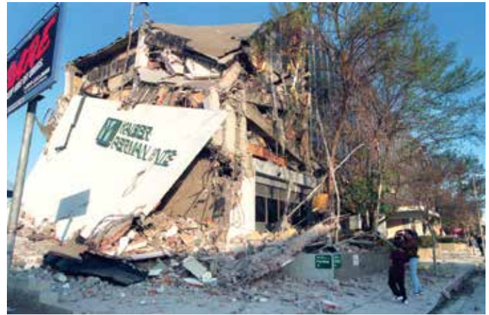
Figure 3. Damage to this non-ductile concrete frame building.
