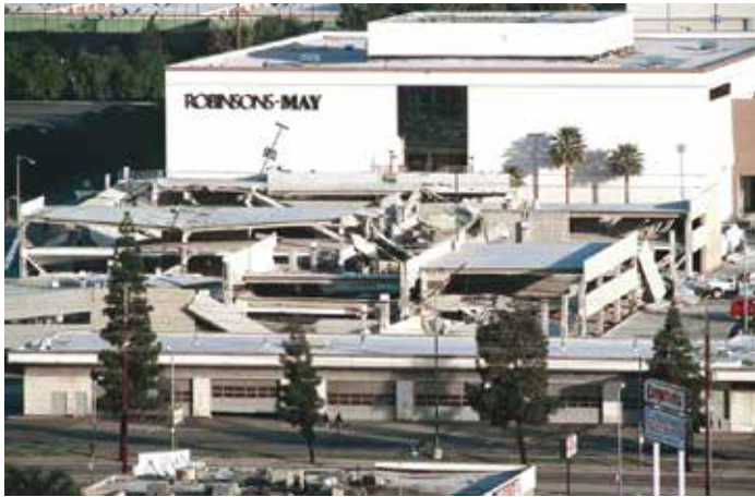
Figure 2. Collapse of the precast concrete parking garage at Northridge Fashion Center.
