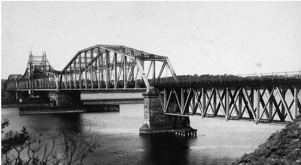
Thames River Bridge.
