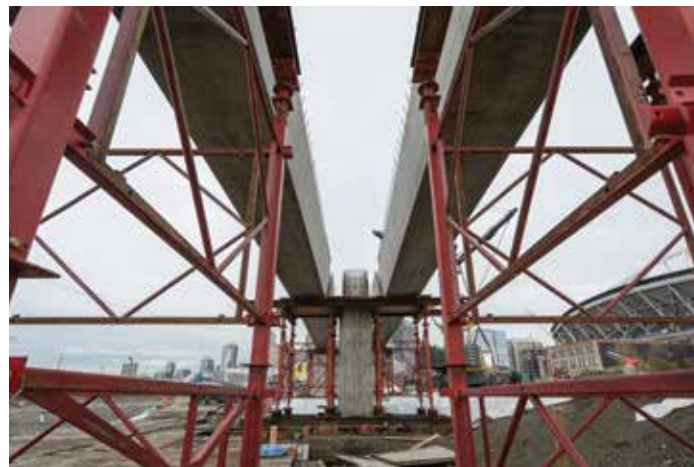
Bridge column with SMA and ECC. Courtesy of Washington State Department of Transportation.
