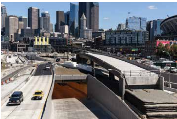
The first seismic resilient bridge in Seattle, WA to incorporate SMA and ECC.
