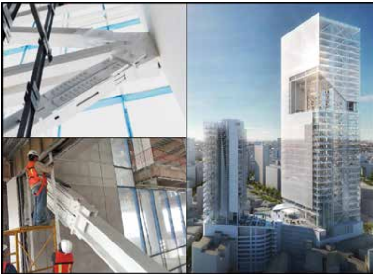
Figure 12. The high-performance Torre Cuarzo tower, with energy dissipation and restoring mechanisms that led to resilient behavior during the 2017 earthquake. Courtesy of Richard Meier & Partners Architects LLP, and Diámetro.
