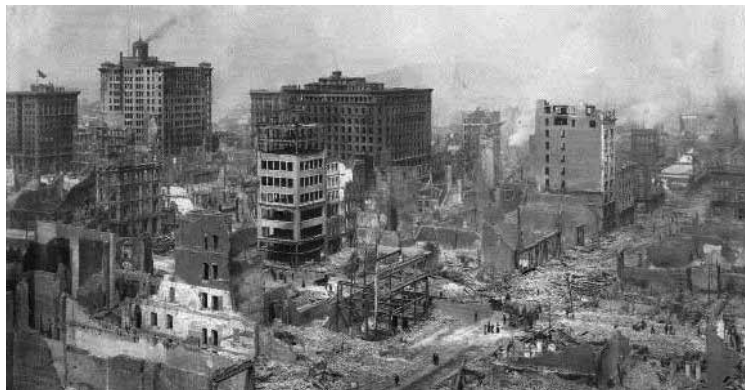
Figure 1. Early steel frame high rises, sole survivors of the SF earthquake and fire.
