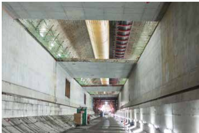
Figure 7. Skip forming for upper slab of interior structure.
