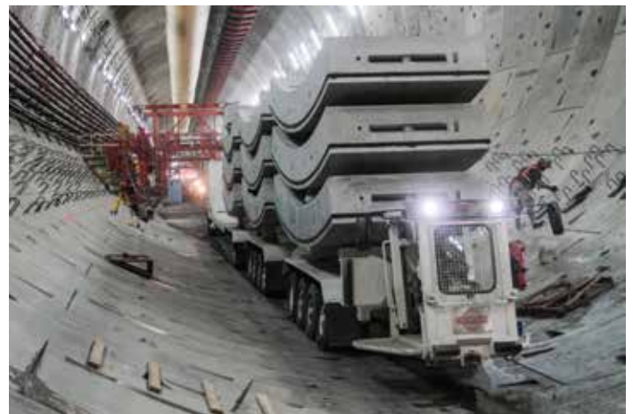
Figure 8. TBM delivery during TIS construction.
