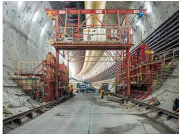
Figure 6. Tunnel interior structure corbel construction.
