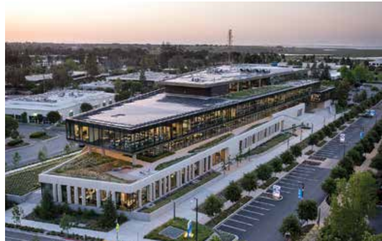
Holmes Structures was an Award Winner for its Intuit project in the 2018 Annual Excellence in Structural Engineering Awards Program in the Category – New Buildings $20M to $100M. Photos courtesy of Jeremy Bittermann.
