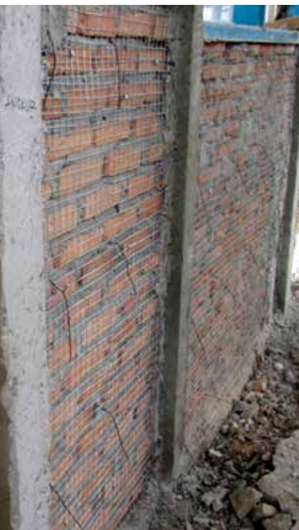
Installation of the mesh plaster overlay during pilot construction.
