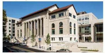
At the University of Connecticut's new Hartford Campus, retaining an essential piece of Connecticut history, the existing Hartford Times Building (Donn Barber, 1920) façade presented unique structural challenges. The façade was repurposed as the framework for a new state-of-the-art facility built
