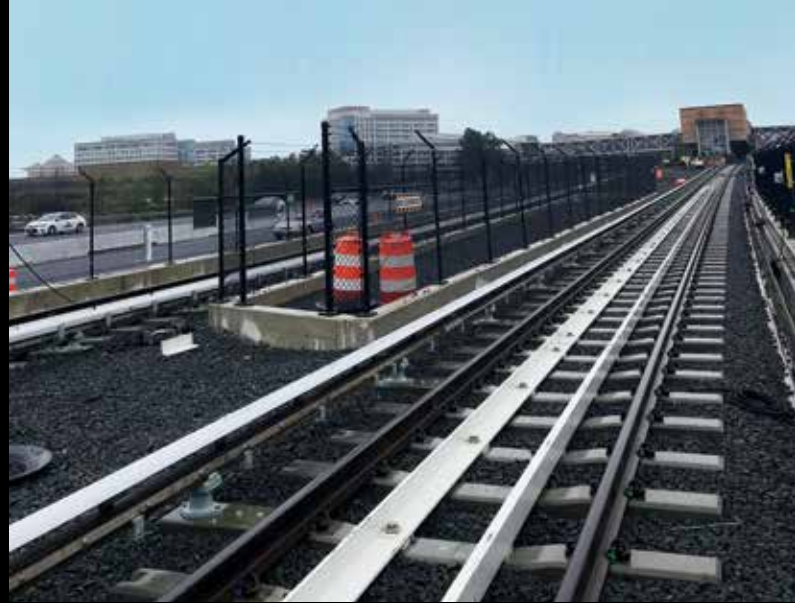
Figure 2. Completed structure in the interim phase.
