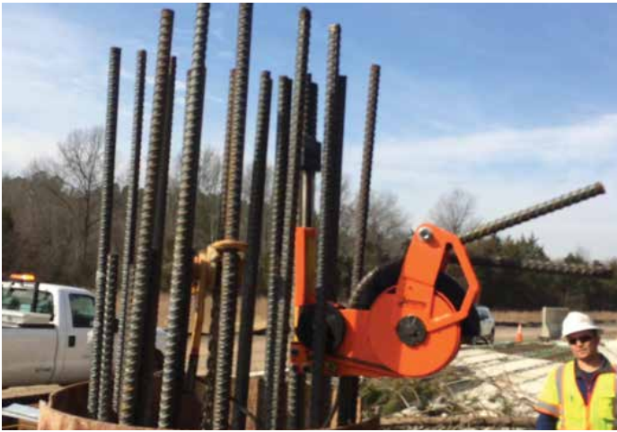
Figure 4. Field bending of bundled #14 reinforcement.
