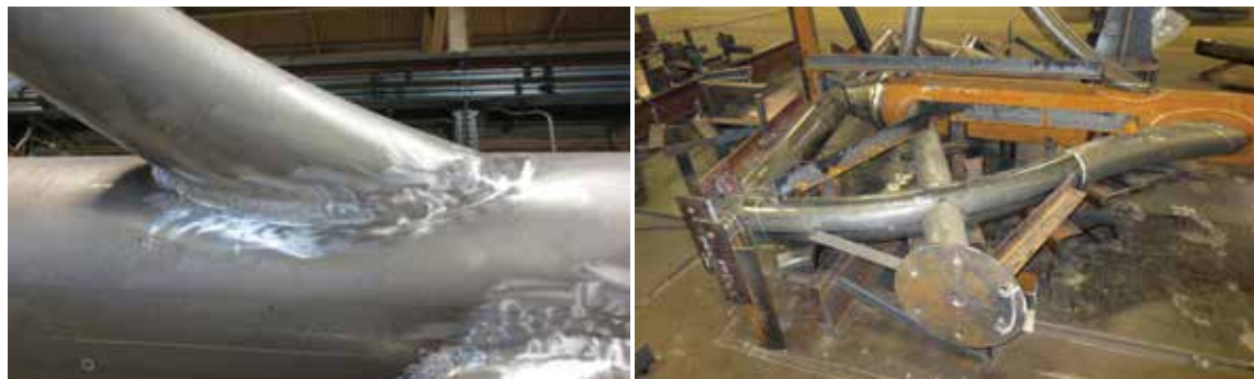
Figure 3. Ground welds (left) and jig for tree columns (right).
