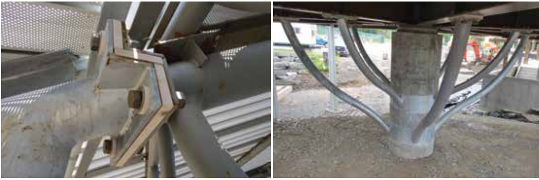
Figure 4. Thermally broken connections at rotunda and atrium.
