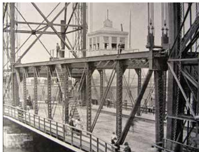
Halsted Street, view of lifting span with a control tower on top of the span.
