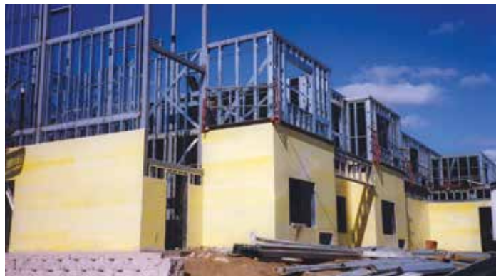
Figure 2. Cold-Formed steel framing with structural wood sheathing.
