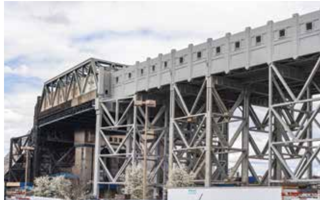
Culver Line Viaduct after.
