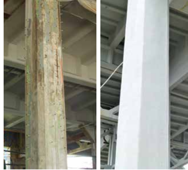
Culver Line Viaduct pillar before. Pillar after.
