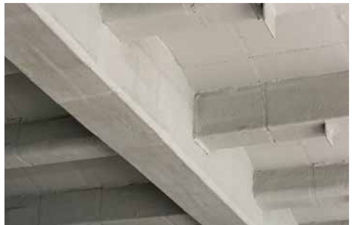
Close up of Culver Line Viaduct.
