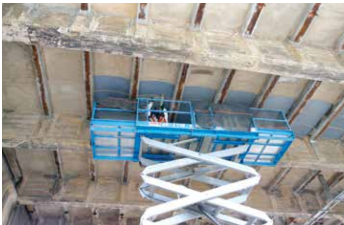
Culver Line Viaduct in progress.
