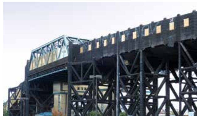
Culver Line Viaduct before.
