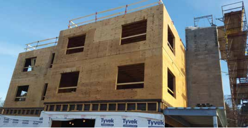
Figure 4. Masonry shaft wall in wood frame building.
