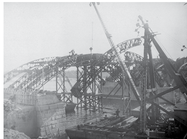
Arch erection in span 7, Springfield side. Courtesy of the Lyman and Merrie Wood Museum of Springfield History.
