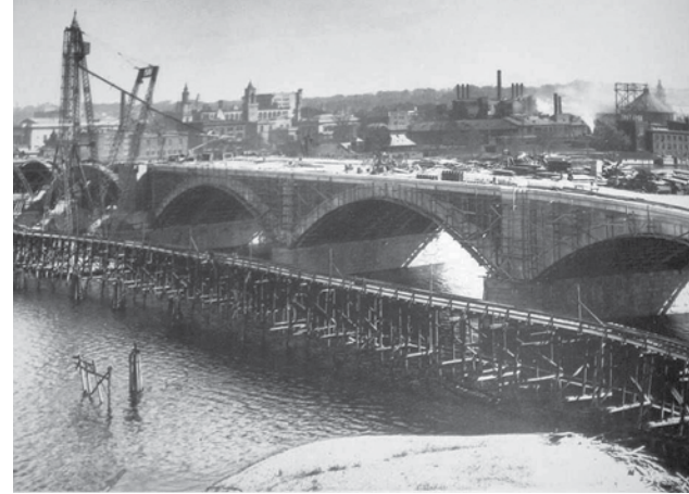
Bridge construction. Concrete hoisting tower (130 feet) shown. Concrete was transported from mixing plant on West Springfield side along a temporary wood trestle 70 feet upstream. Courtesy of the Lyman and Merrie Wood Museum of Springfield History.
