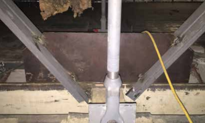
New truss V-Web with temporary hanger rod in the foreground.
