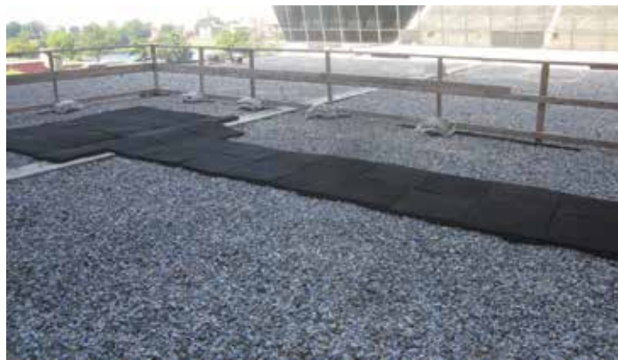
Roof before renovation.
