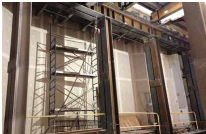
Final structural framing for McKim wall. Johnson concrete walls removed.
