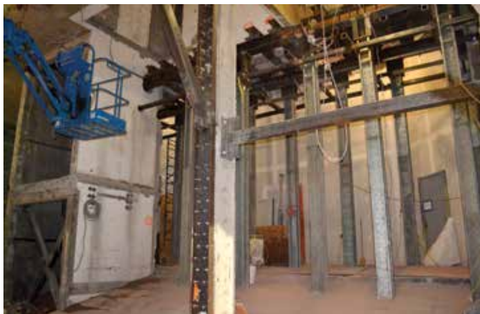
Temporary shoring with McKim wall removed. Johnson concrete walls left.
