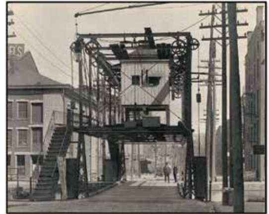
Hotel street bridge after reconstruction.
