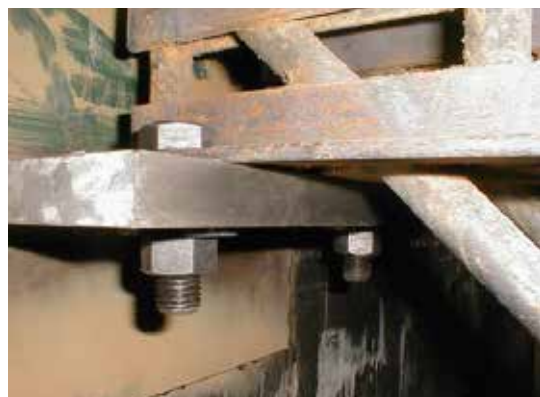
Figure 1c. Floor end unrestrained (resting) on support for unrestrained test.
