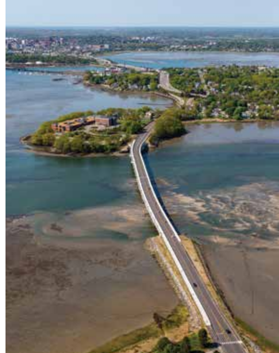
Geotechnical peer-reviewed design-build bridge, Martin's Point Bridge Portland-Falmouth, ME. Courtesy of Dave Cleaveland, Maine Imaging.
