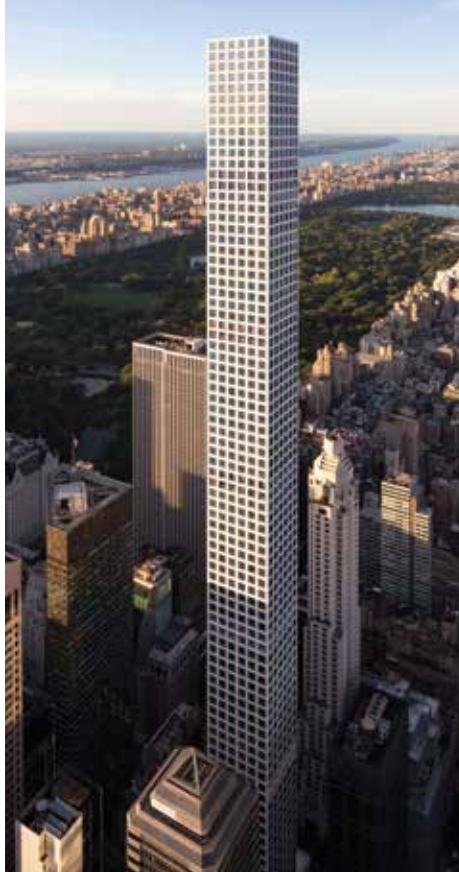
Figure 2. Overview of 432 Park Avenue after completion of construction.
