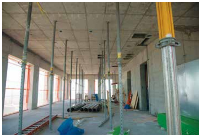
Figure 1. Detail of the open floor layout during construction.
