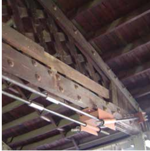
Figure 2. Bottom chord of bowstring truss retrofitted by installing steel tension rods along the span of the truss (left). The steel bracket at the end of the truss (right) transfers the force from the top chord to the new steel rods.
