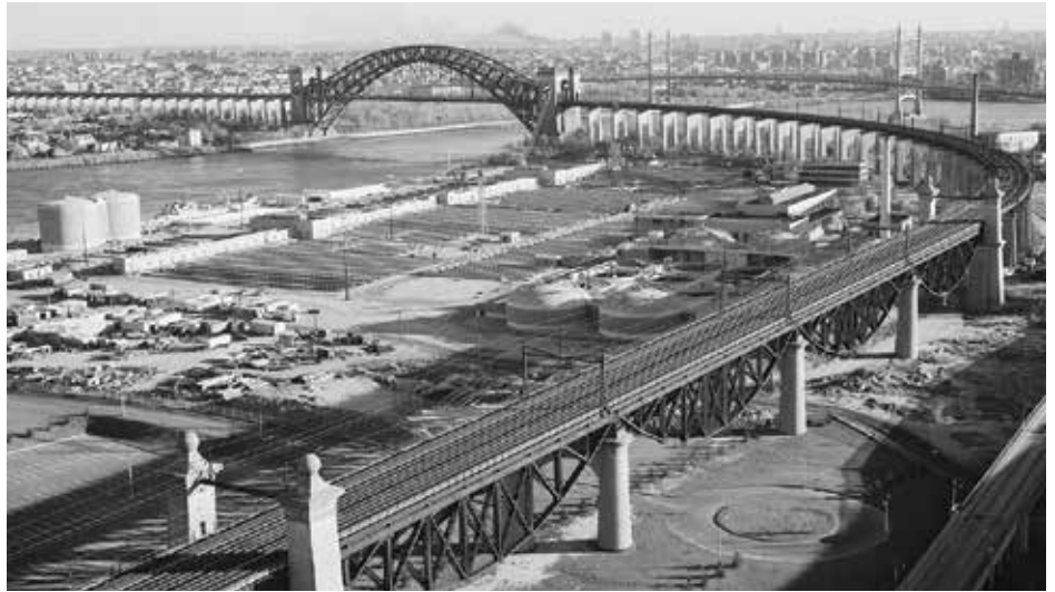
Hell Gate Bridge, Viaduct, Little Hell Gate Bridge (inverted bowstrings) foreground. Courtesy of HAER.
