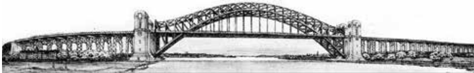
Profile of Hell Gate ( Engineering Record ) with original steel approach towers and spans.
