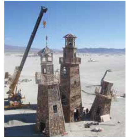
Figure 2. Installation of towers onto wedges.
