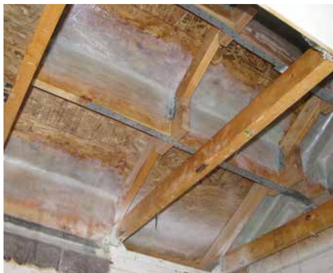
Typical installation of FRP in a wood roof system.
