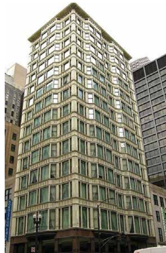
Figure 1. The Reliance Building, Burnham and Root/Atwood. Example of an early steel frame terra cotta clad building. Courtesy of TheArchitecturePost.com .
