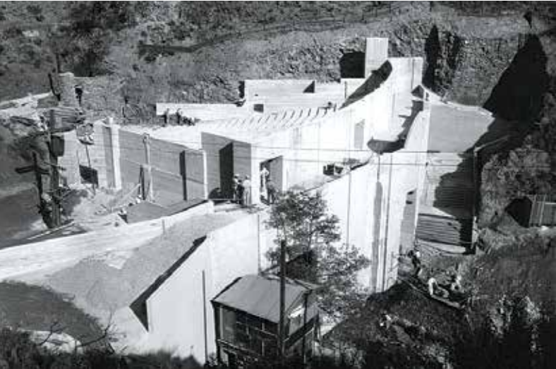
Figure 1. The theater reconstruction out of reinforced concrete (1931). Courtesy of the Los Angeles Public Library Photo Collection.
