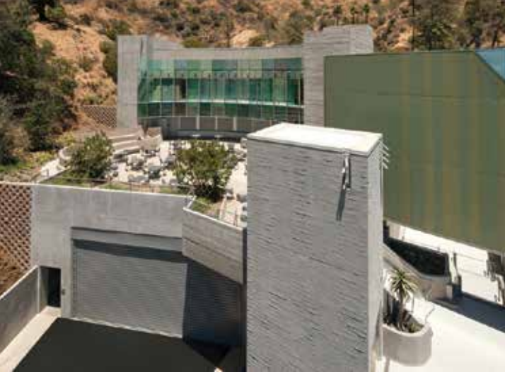
Figure 5. The new Ford Terrace building on the north side of the amphitheater. Courtesy of Tom Bonner Photography.
