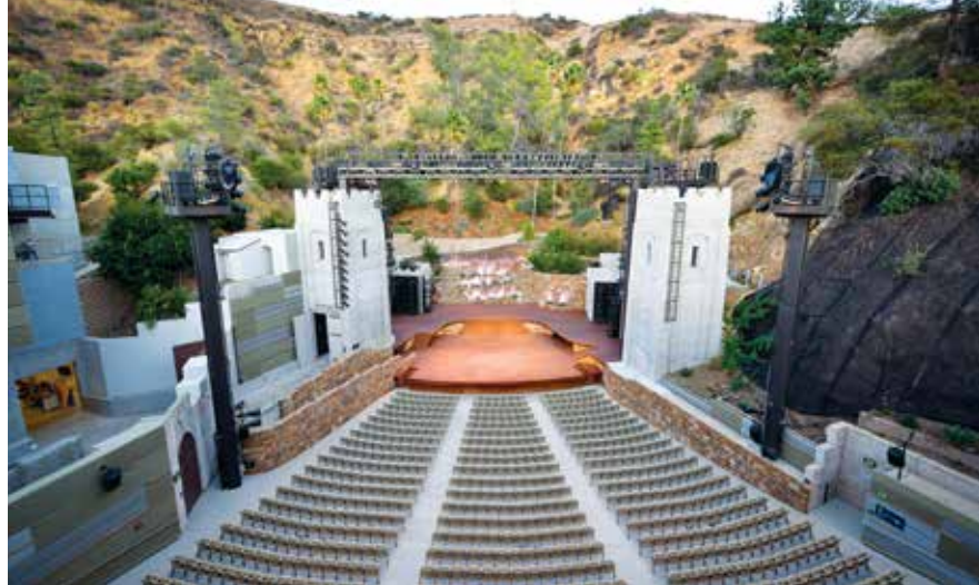
Figure 6. Renovated John Anson Ford Amphitheatre.
