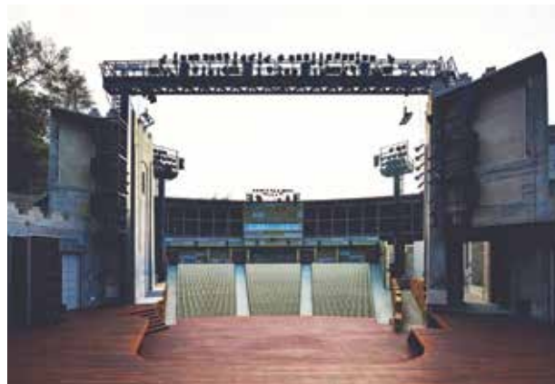
Figure 4. New sound wall and control booth behind the amphitheater.
