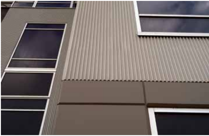
Concrete tilt-up wall panel with various form liners and reveals. Innovative brick systems were also used to cast thin brick into some of the tilt-up wall panels.
