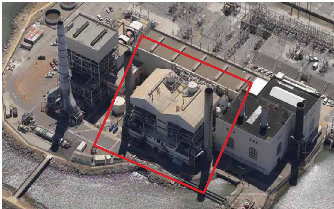
Figure 1. Aerial view of power plant (boiler outlined). Courtesy of Pictometry.
