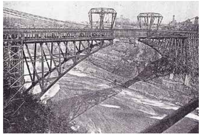
Erection under Roebling Suspension Bridge.
