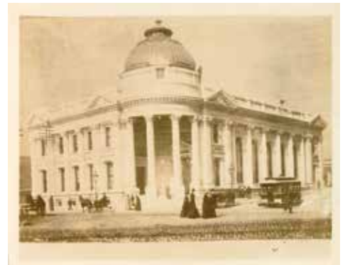
Figure 1. Hibernia Bank Building in 1894, before the addition. Courtesy of San Francisco History Center, San Francisco Public Library.
