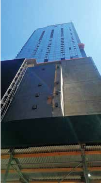
Topped out and clad.
