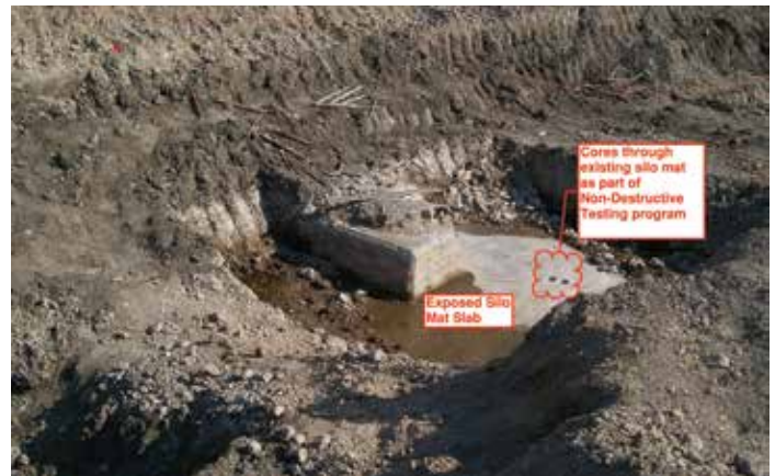
Figure 5. Existing silo mat foundation. Courtesy of LAN.
