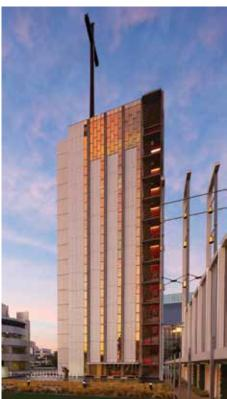
plates. The performance-based design strategy limited major construction activities to four of the tower's thirteen floors, which proved to be far more efficient and less disruptive than a traditional retrofit strategy.
