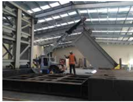
Figure 5. Assemblage of test frame in the warehouse.
