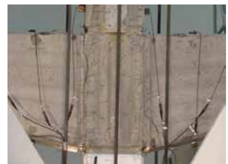
Figure 8b. Specimen damage after cyclic testing.
