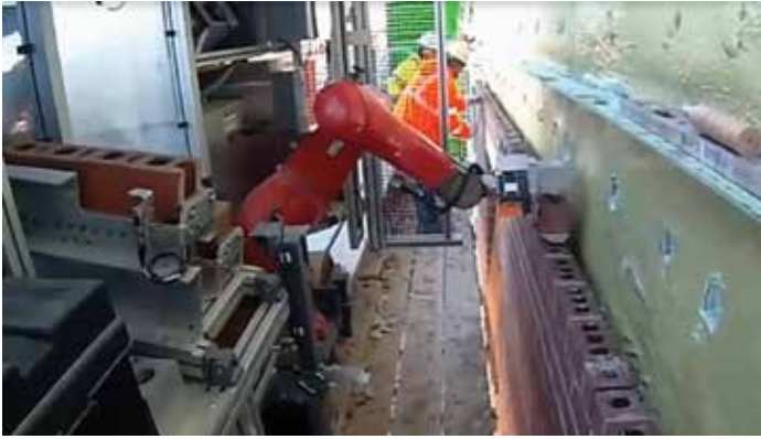
Figure 3. Robot laying a brick wall.
