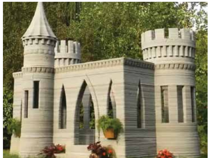
Figure 5. 3D printed concrete castle.
