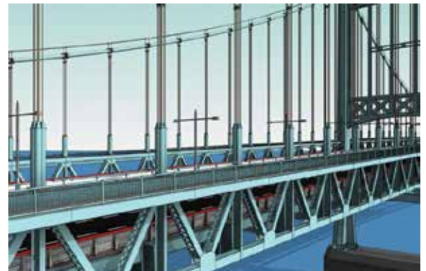
Figure 5. Shallow Fascia girder.
