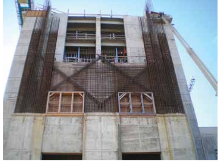
Diagonal reinforcement at the special shear wall.
