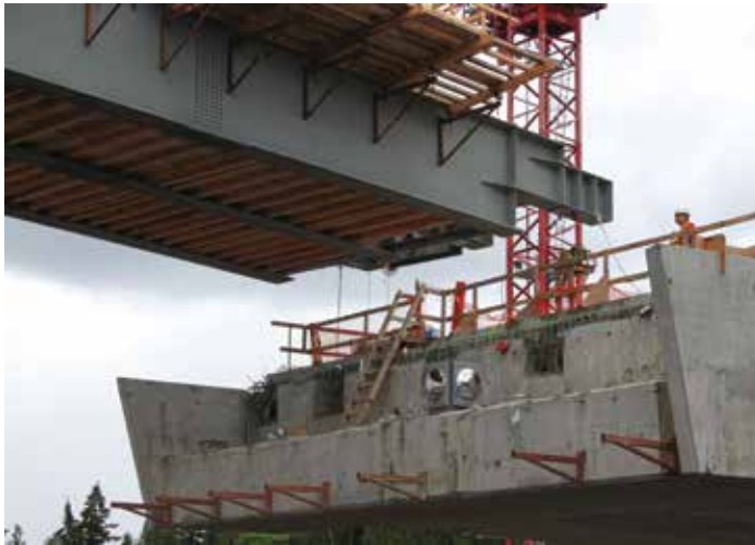
Figure 4. Girders being erected over the trailer hitch.
