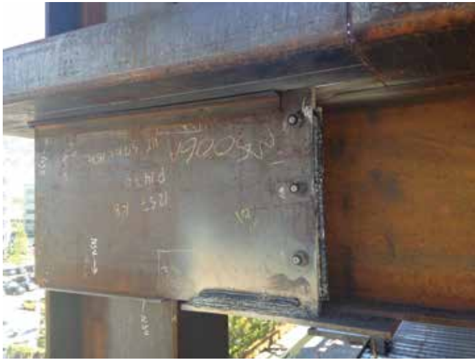
Figure 2. SidePlate connection.
