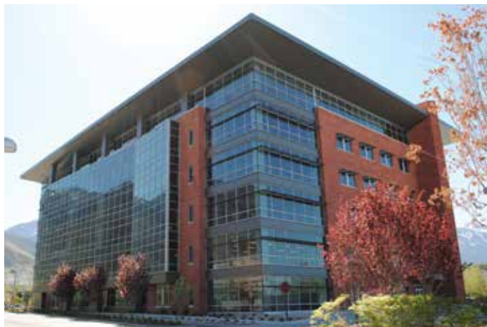
Figure 6. Cut sandstone façade and full height windows.
