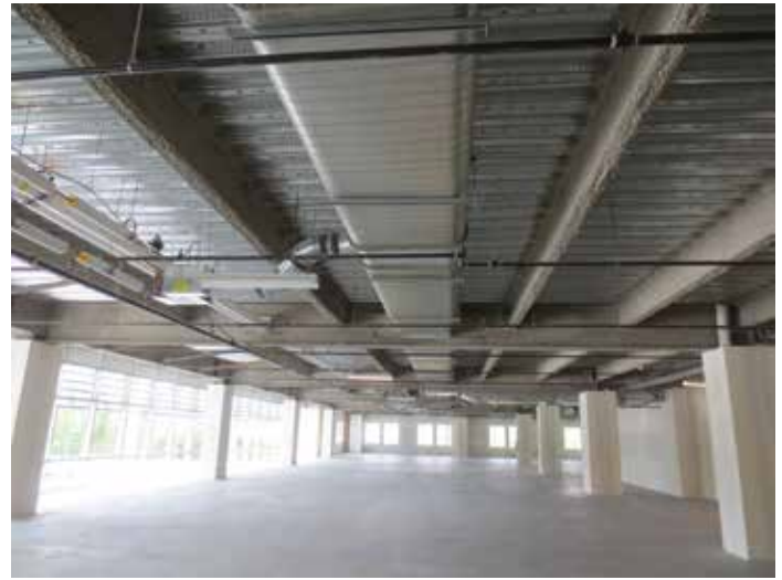
Figure 3. Steel girder web openings.
